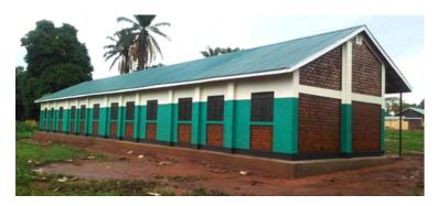
**Classroom block and latrines at Baguya Primary School:** Construction of a 1x4 CRB with wooden furniture and two 5,000L rainwater harvesting tanks in Maridi is complete. Construction of latrines for girls (with washrooms), boys and teachers has commenced. All structures are built using ISSB.
