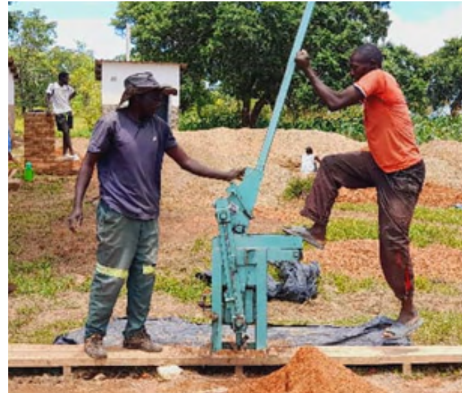
Moulding ISSB bricks, Zambia
