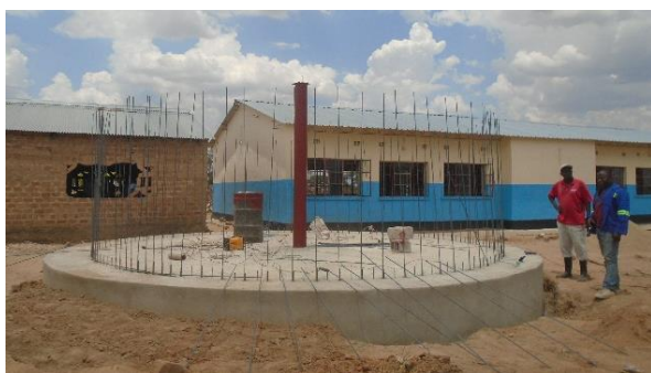
Rainwater harvesting tank – under construction and completed
