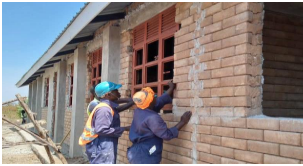
Construction of CRB
