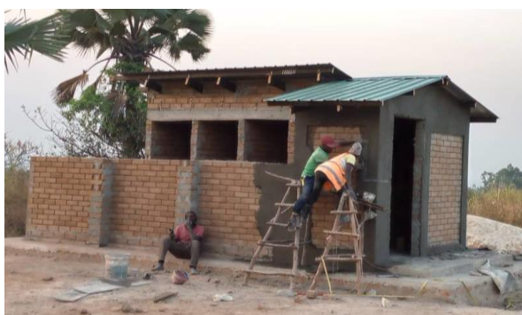
Construction of latrines
