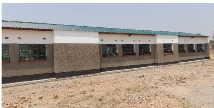
Completed classroom block
