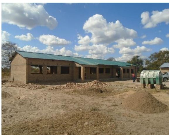
Classroom block under construction
