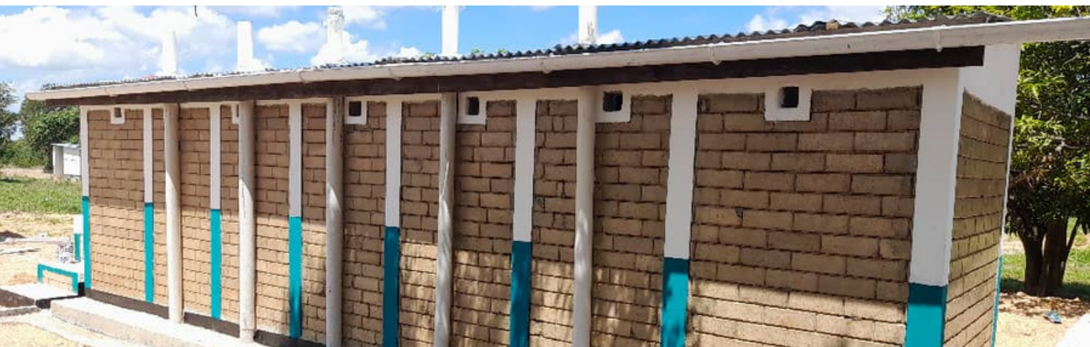
Completed latrines at Tara Primary School
