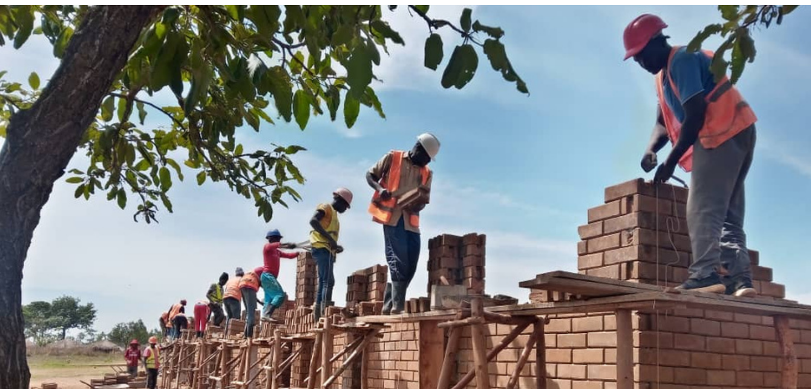
Construction progress at Busia Primary School, Koboko District
