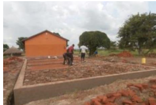
Starting the Foundations
