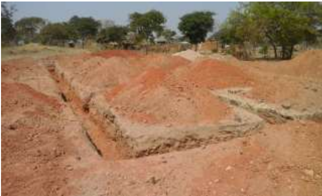
Digging foundations, August 2018
