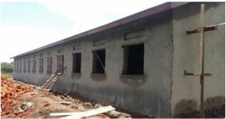
Figure 3: The walls are plastered
