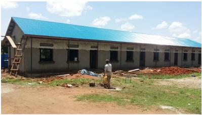
Figure 4: The completed roof on Haddow Secondary School
