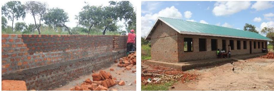
Caption: Progress of the construction at Aditiru Primary School
