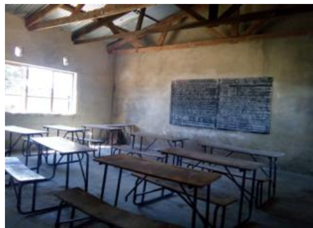
Before: inside of classroom block
