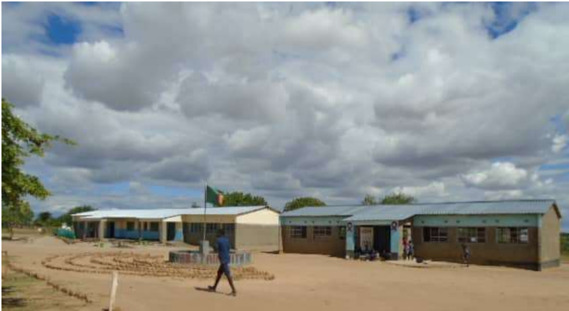
New block on the left with 3 classrooms, older block on the right with 2 classrooms.
