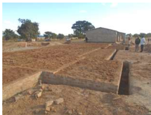
Slab level, July 2018
