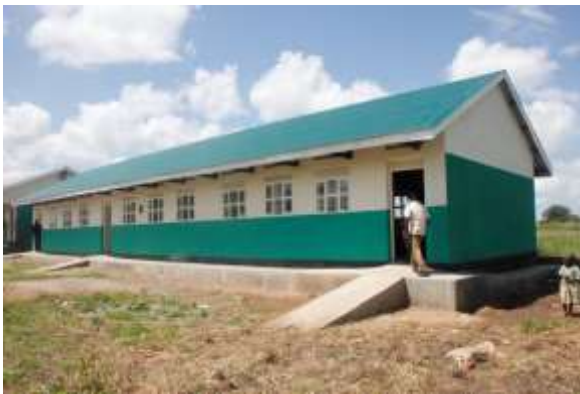
New classroom structure
