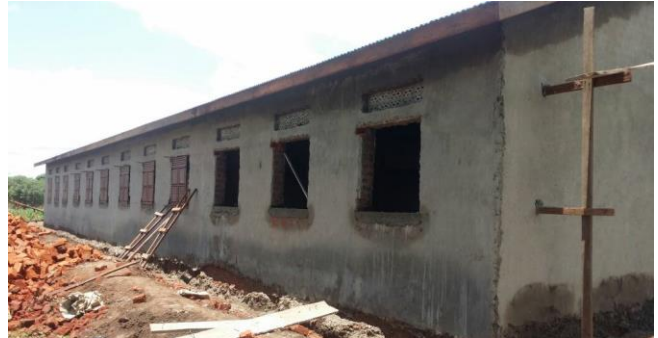
Figure 3: The walls are plastered
