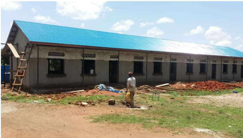
Figure 4: The completed roof on Haddow Secondary School
