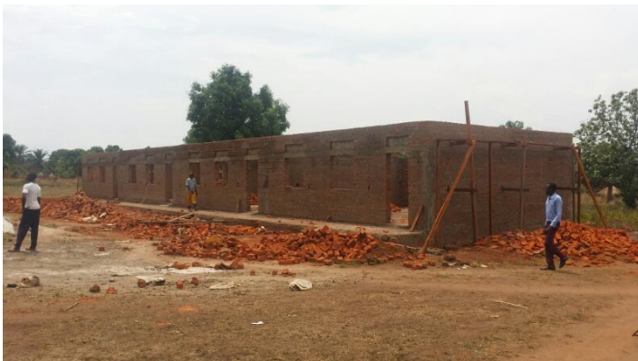
Figure 2. Completion of the wall
