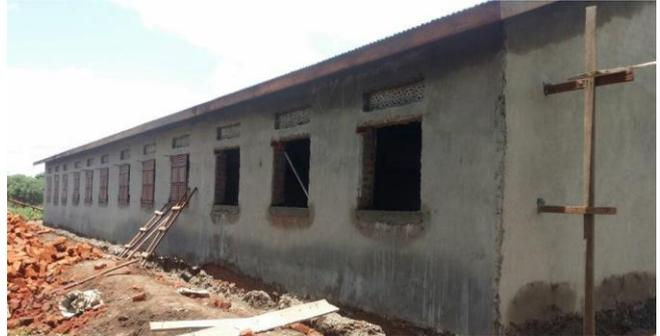
Figure 3: The walls are plastered
