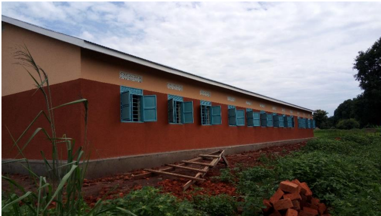
The finished four-classroom block at Hadow Secondary School, Maridi
