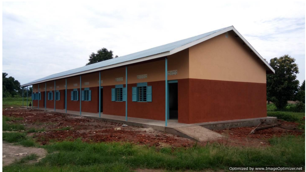
Figure 5: The completed front of school only the groundworks to complete
